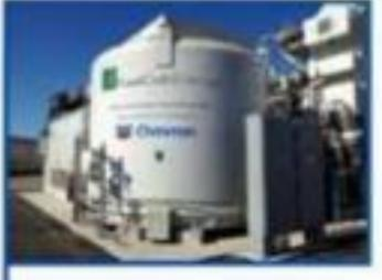
2 MW, 4 MWh Advanced BYD Energy Storage System
