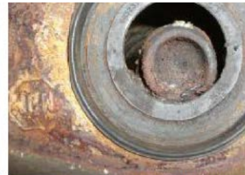
Corrosion inside the brake housing
